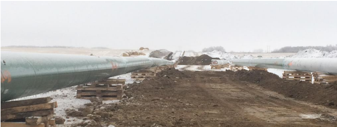
Montgomery Creek 714 + 600 – product Pipe strung along right of way
