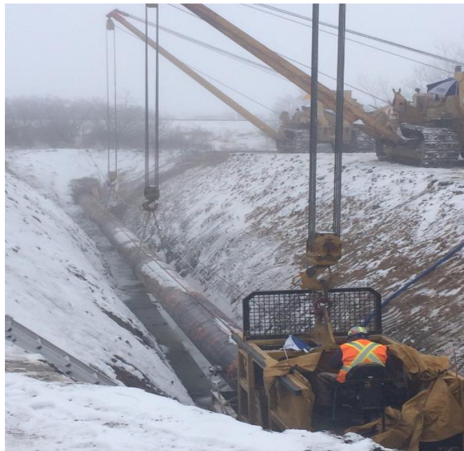
795 + 877 Cradle bore under the tracks
